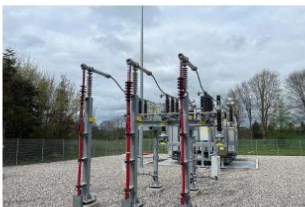
Figur 9. Illustration af transformerstation.
